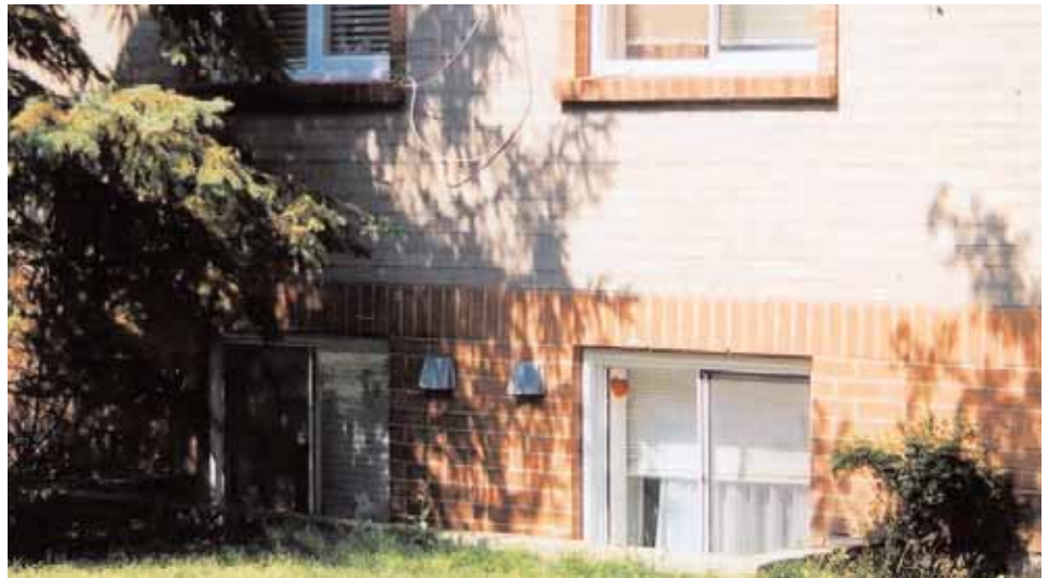
Large wells permit big basement windows, improve natural light and ventilation and may facilitate exiting Photo by Barry Craig
